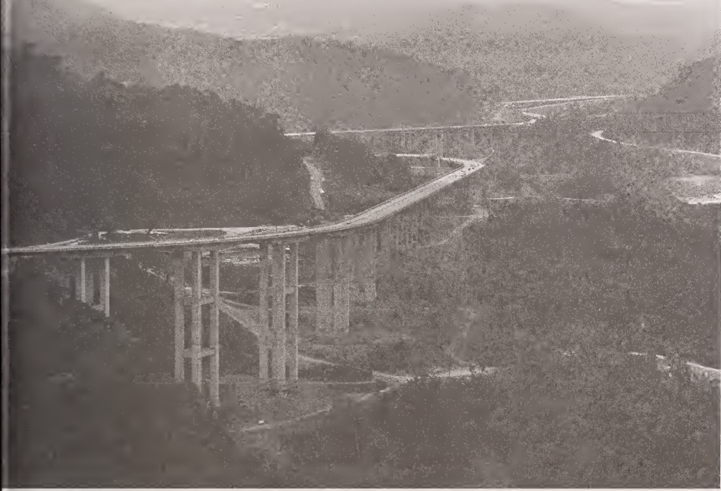
The three-lane Immigrants Highway climbs 700 meters from the Atlantic to the plateau in a continuous grade marked by a spectacular series of tunnels and bridges. Courtesy Inter-American Development Bank, Washington
